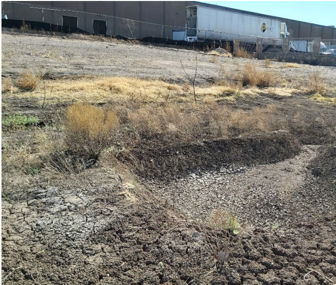
PHOTO NO. 15: General southwest view of existing ponding area slope conditions.
