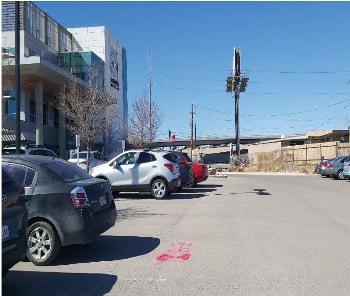
PHOTO NO. 7: General north view of box culvert route and existing conditions at vertical boring B-3.
