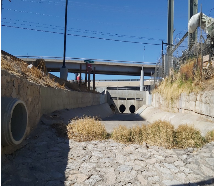
PHOTO NO. 1 General north view of existing concrete channel conditions.
