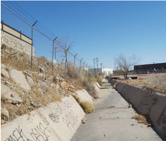
PHOTO NO. 3: General southeast view of existing concrete channel conditions.
