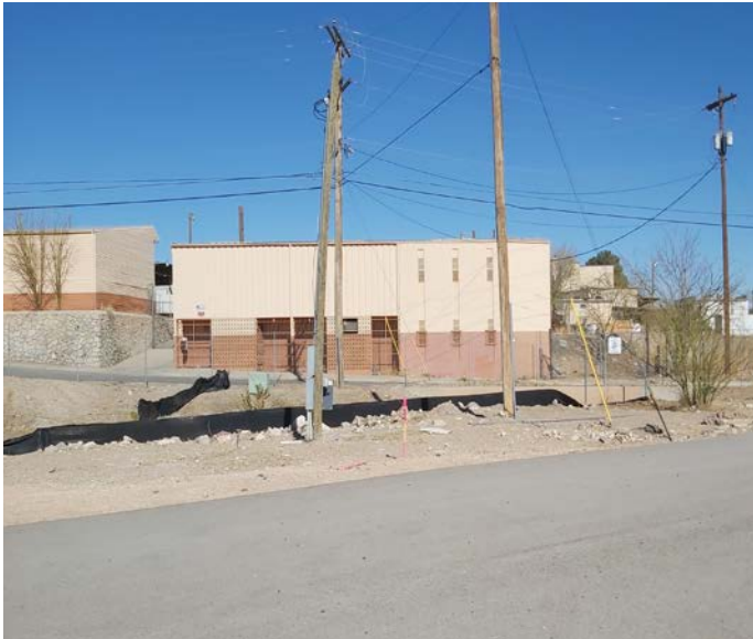
PHOTO NO. 11: General east view of box culvert route and existing conditions at vertical boring B-7.
