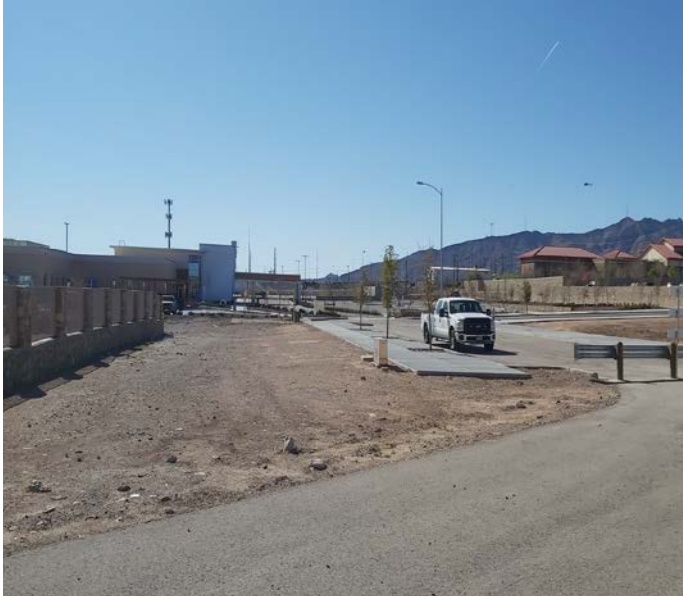
PHOTO NO. 5 General west view of project site existing conditions along future box culvert.
