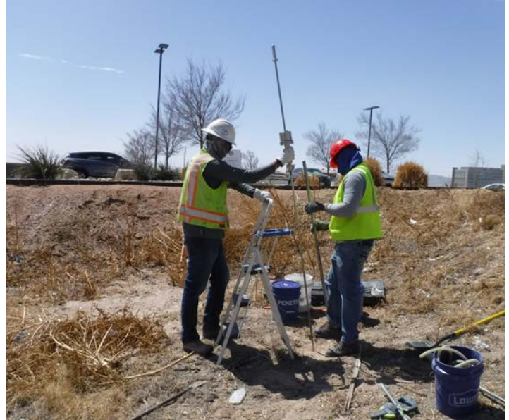
PHOTO NO. 18: General view of our DCP test at HAB-2 / DCP-2.
